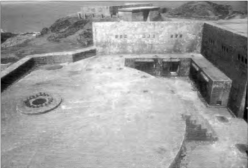
Fig. 11 Interior of Second World War gun house E2 showing the attachment for the naval 6-inch gun and ammunition lockers. The other gun house (E1) can be seen beyond with its crew rooms to the rear and the remains of the supports for the plastic armour roof; photo Somerset County Council
