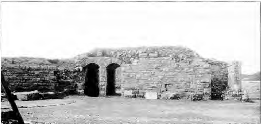
Fig. 10 The south side of the artillery store. The racer rail for the 'A' pivot G6 can be seen on the left; photo SANHS collection lantern slide
