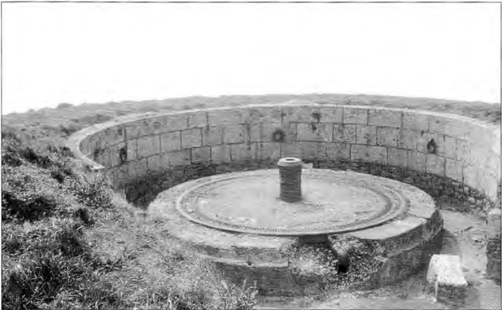
Fig. 12 Gun position G4 in the early 20th century showing the experimental alterations to the 'C' pivot. The ground has been lowered outside the racer rail, revealing the foundations of the parapet wall, and a toothed ring added for traversing the gun; photo SANHS collection
