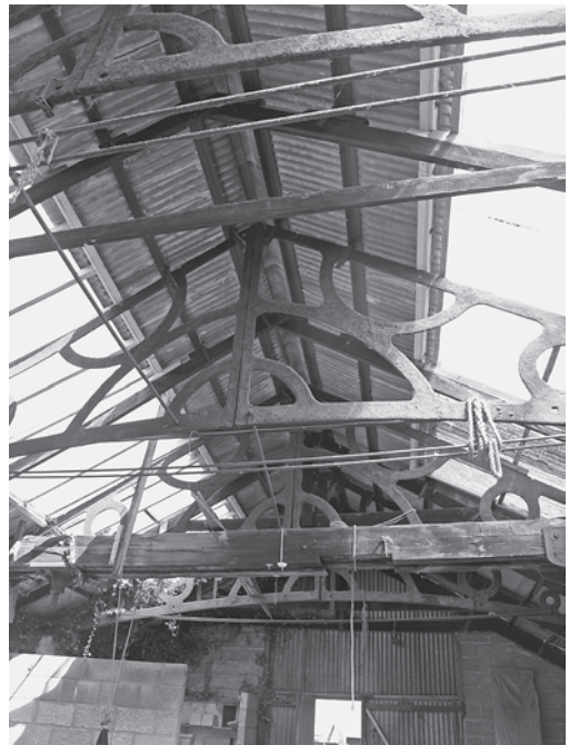
Fig. 4 Watchet foundry, cast iron trusses (photo Patrick Stow)
