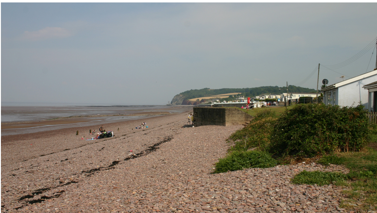
Figure 3.11: Blue Anchor Bay. The only surviving section post of some 23 constructed in the first phase of coast defences in the summer of 1940. The post has 11 loopholes and is sited to cover the beach with rifle or machine-gun fire along the high water line. There is a pit for a light AA machine-gun in the centre of the roof. SHER 35367, Listed Grade II in 2010. The beach defence gun was sited in the woods, just below the horizon (David Dawson, 2010).
