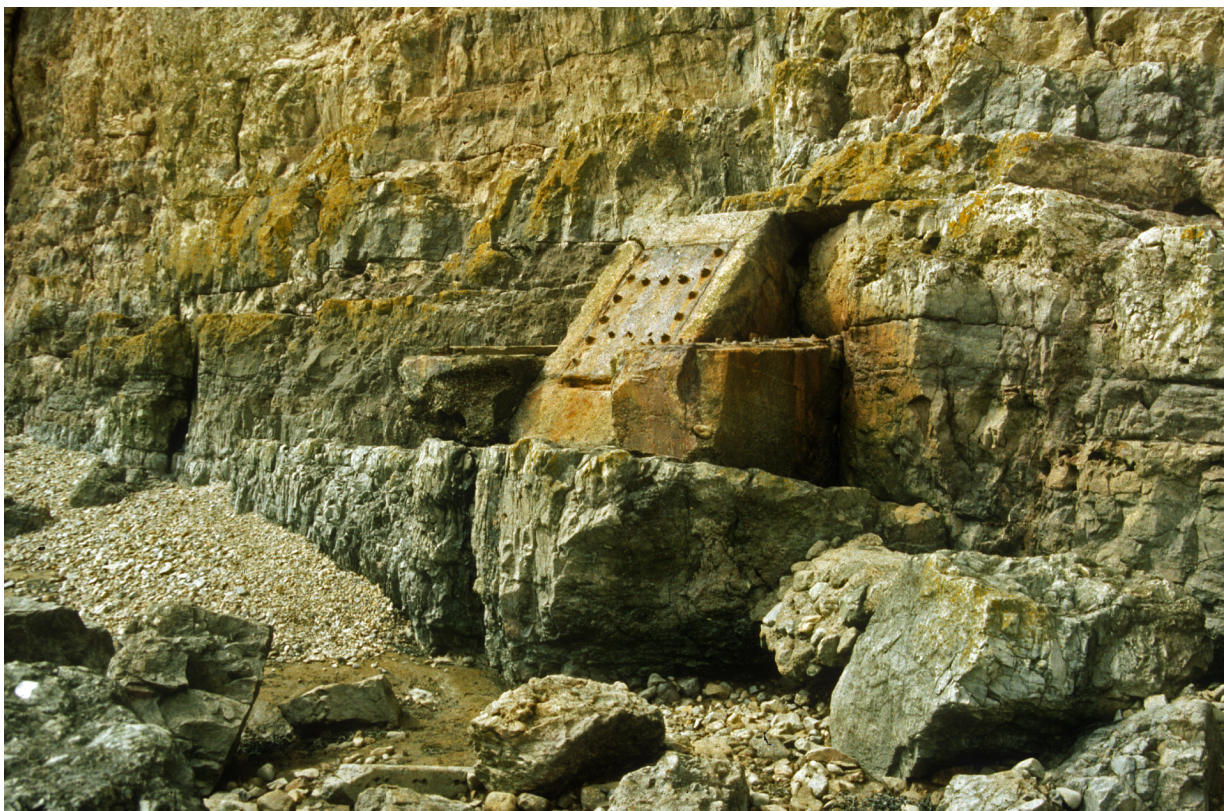
Figure 6.12: The remains of some of the steel fixings to the rocks on the beach at the foot of the cliffs of Brean Down (Somerset County Council HER, 1995).
