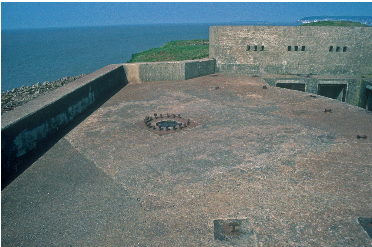
Figure 4.4: Remains of one of the two 6-inch gun emplacements at Brean Down. Compare this with the contemporary painting of an identical emplacement on Steep Holm on the cover of this volume. The ring bolt for mounting the gun lies in the centre with the cut-off remains of the supports for the plastic armour roof around it. Birnbeck Pier can be seen in the distance (Somerset County Council HER, 1995).
