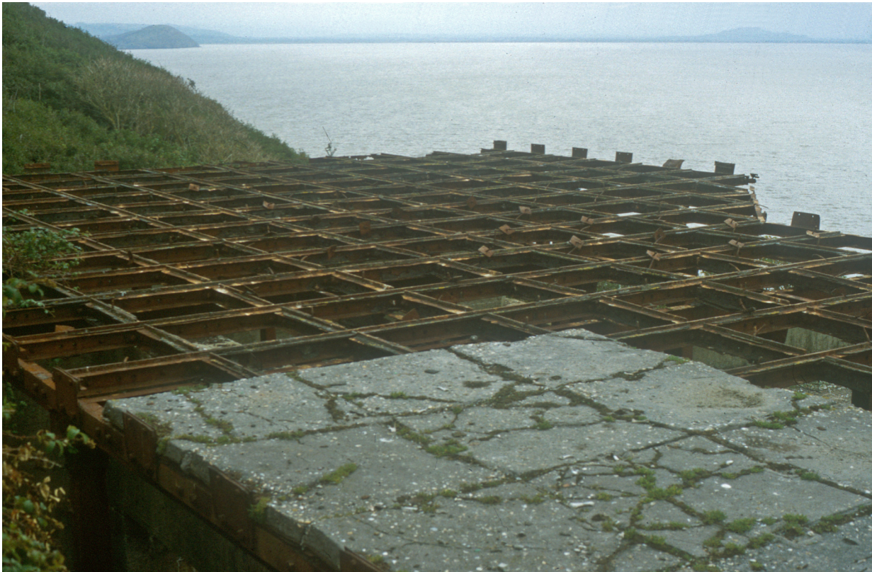
Figure 4.6: Sections of surviving plastic armour roof at Steep Holm South Battery. Most of the armour has been removed to prevent the collapse of the steel frame. Brean Down can be seen in the background (Chris Webster, 1995).
