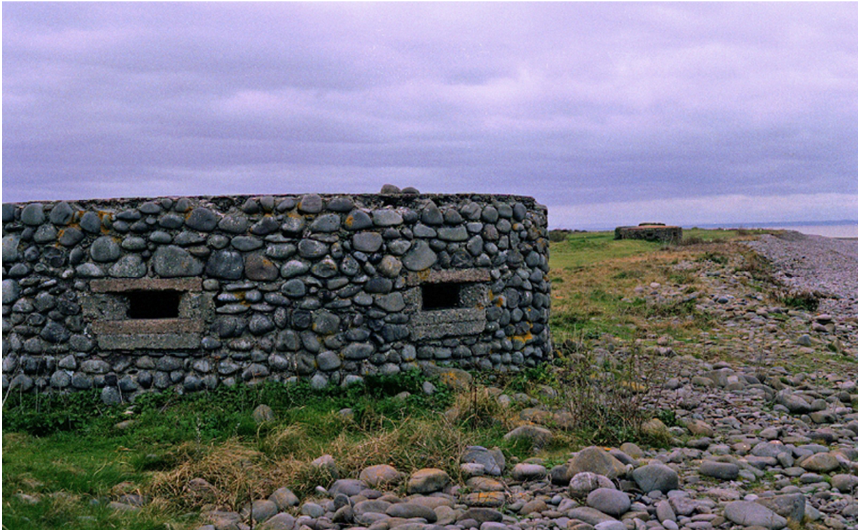
Figure 3.10: Pillboxes camouflaged with beach pebbles on the coast north of Dunster Beach. SHER 35362, 35363 (Timothy Dawson, 2002).
