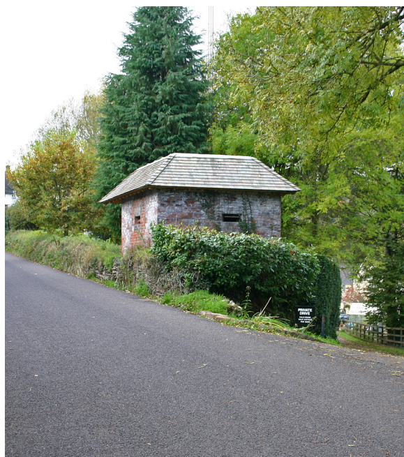
Figure 3.12: Pillbox at Vale House, Roadwater, with camouflage roof reconstructed in 2008 by Exmoor National Park Authority. It was built in 1940 to cover an anti-tank roadblock closing routes towards the west Somerset coast for German troops landed by air on the Brendon Hills. ExHER MSO12289, Scheduled Monument 35320 (David Dawson, 2009).
