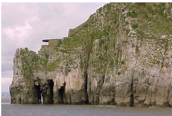
Figure 4.5: Coast Artillery searchlight on Steep Holm. The searchlight was sited in a low position to maximise the area of sea swept by the narrow beam (David Hunt, 2001).
