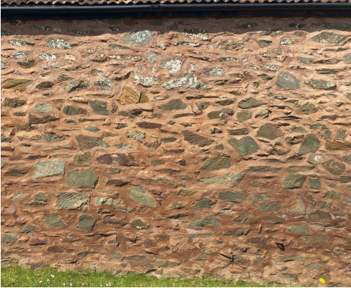
Fig. 9 Former barn wall adjoining Plainsfield Court showing use of Cockercombe Tuff rubblestone laid randomly with other blocks of Hangman Sandstone and Ilfracombe Slates (ST 19560 36582).
