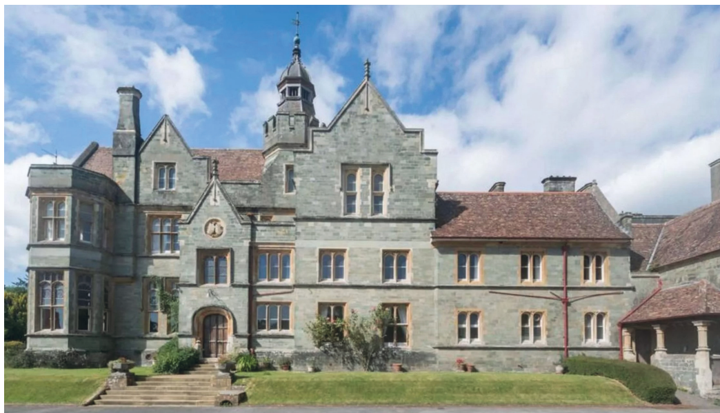
Fig. 6 Quantock Lodge (ST 18797 37542), near Over Stowey. Grade II listed. Built in 1857 (additions made in the 1860s) in Free Tudor style using dressed ashlar blocks of Cockercombe Tuff with Bath Stone dressings.
