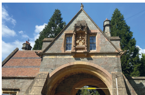
Fig. 7 Quantock Lodge Gatehouse (ST 19354 37371), near Over Stowey, formerly part of Quantock School. Grade II listed, built in 1857 of dressed blocks of Cockercombe Tuff with Bath Stone and Helmsby Sandstone ('Otter Sandstone') dressings.
