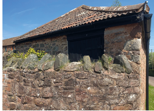
Fig. 10 Entrance wall at Plainsfield Court with Cock and Hen arranged capping slabs of Cockercombe Tuff atop blocks of Hangman Sandstone and Ilfracombe Slates (ST 19557 36571).
