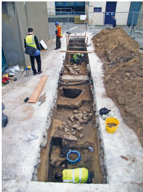
Fig. 6 The 2008 evaluation trench at the School of Science and Art. Facing S
