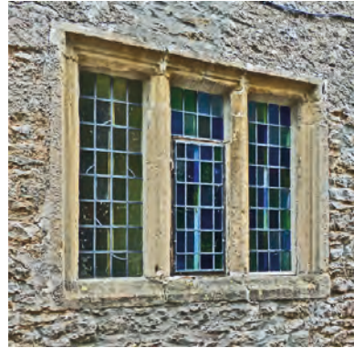
Fig. 5 Window at house No. 11
