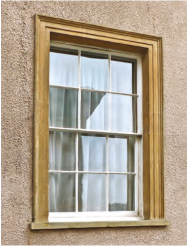
Fig. 4 Exterior window architrave to Coombe House (No. 15)
