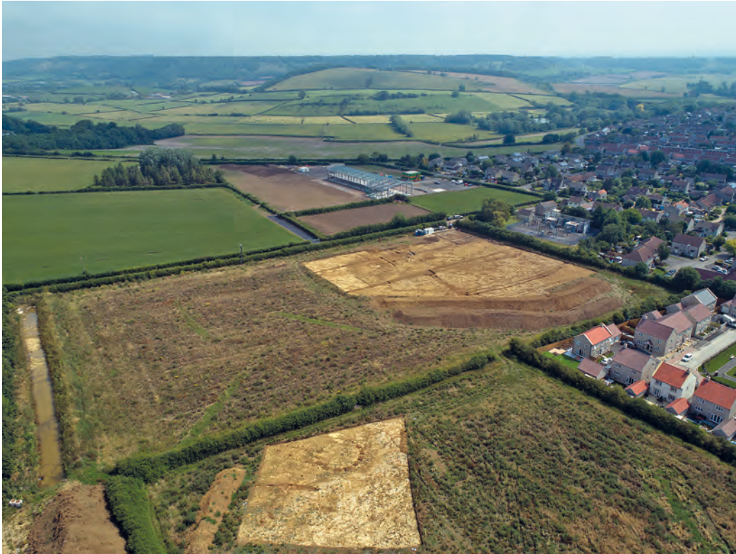
Fig. 3 Aerial view of the site, looking north-east with the new Somerton Primary School under construction beyond
