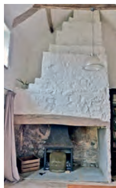
Fig. 4c Godney, Lower Godney House, Annex fireplace with single Lias orthostatic jamb at right
