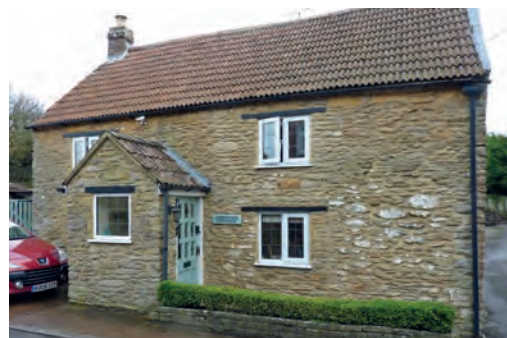
Fig. 3 East Coker, Ebenezer Cottage, Front elevation with windows under timber lintels
