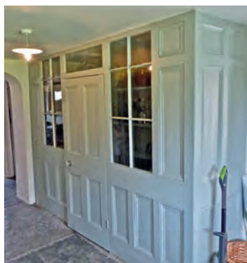
Fig. 4b Godney, Lower Godney House, Panelled and part-glazed cupboard in stair hall
