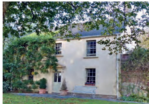
Fig. 2 Coleford, Lydford Farm, South elevation showing bracket and pedimented entrance
