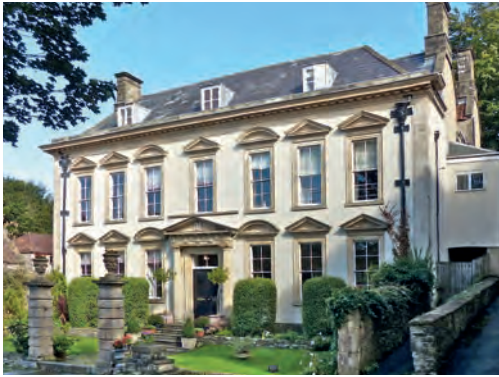
Fig. 5a Shepton Mallet, Bowlsh House, Classical west front with dormers in the hipped roof
