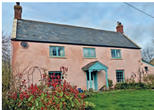
Fig. 4a Godney, Lower Godney House, Rendered south elevation with replica sashes on ground floor
