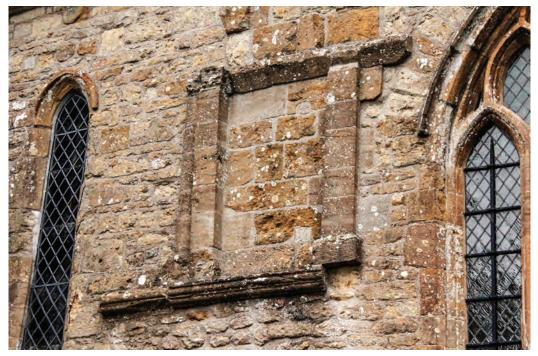
Fig 12 Detail of the engaged column positioned adjacent to a pilaster on the south chancel wall
