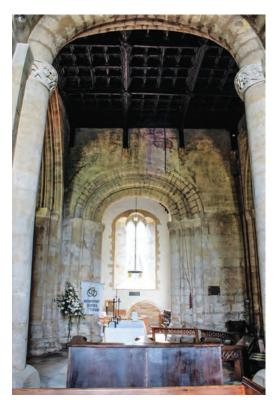
Fig. 8 South crossing arch showing the wider western wall at the location of the external stair turret
