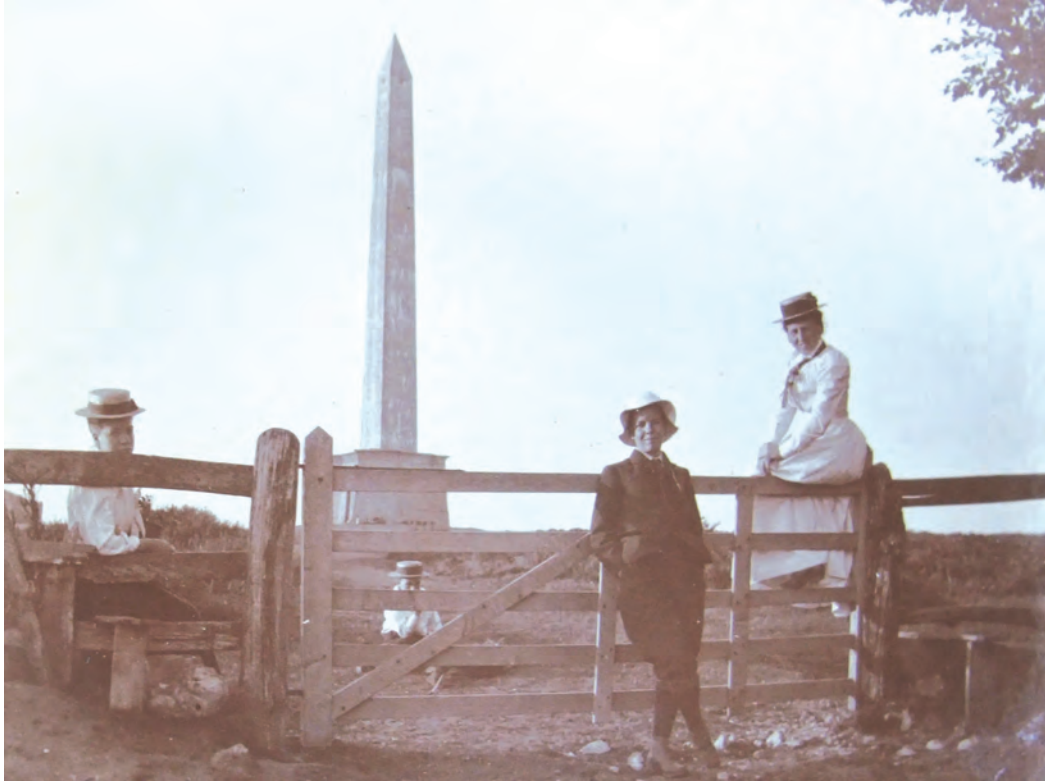
Fig. 6 Enjoying the Monument in 1900/01. The group are posed at the gate and former stile leading to Monument Farm and an accompanying photo suggests they had arrived by bicycle. Staining from washed out lime mortar can be seen on the shaft of the Monument. Reproduced courtesy of SHC
