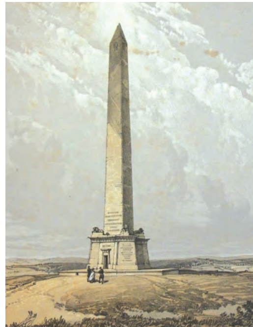
Fig. 4 'Proposed design for the restoration of the Wellington pillar, Wellington. Messrs Goodridge Architects, Bath'. Lithograph. A copy is held by SHC
