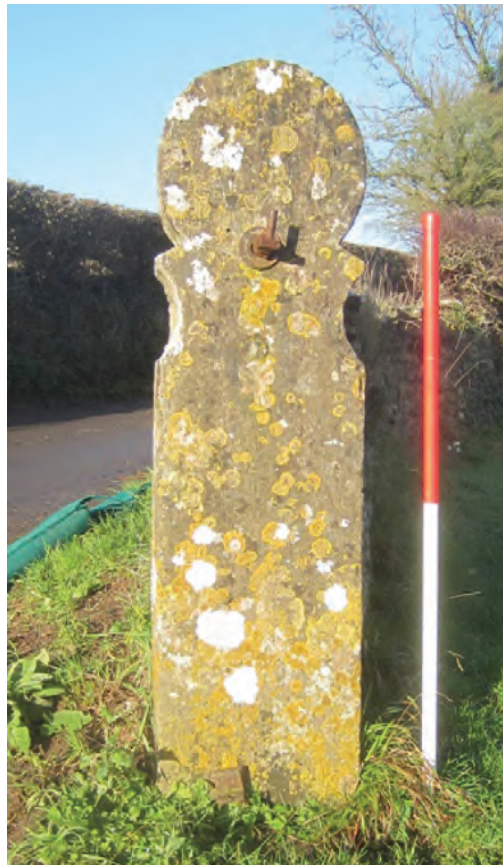
Fig. 4 Nineteenth century Draycott stone gatepost at Old Ditch Farm, Lynch Lane, Westbury-sub-Mendip
