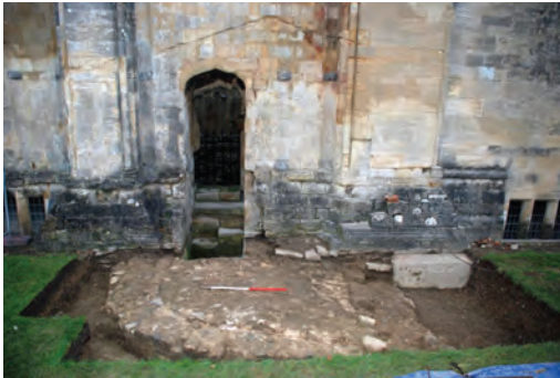
Glastonbury Abbey: Excavation of the vault and wall tops associated with the early 19th-century restoration of the well house, looking north. The angled scars for the medieval gabled roof are also visible.
