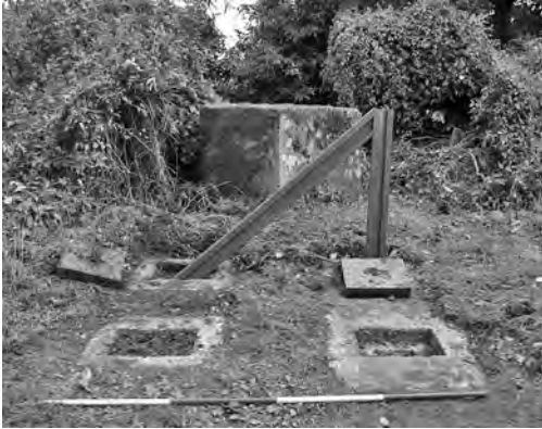
Fig. 1 Part of the Second World War road block exposed at Dillington Drive with a replica bent rail (made by Brian and Chris Perry) showing how the sockets would have been used. One of a line of concrete blocks preventing access around the site, the roadblock is visible in the rear (Photo Somerset County Council)
