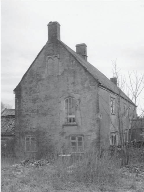
Fig. 2 Rookery Farm, north-facing gable
