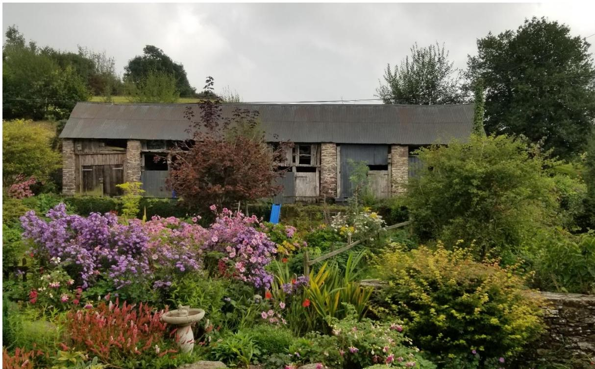
*The Linhay. This traditional farm building was in extremely poor condition a few years ago. The land at the rear of the building was pushing it forward and the whole thing was in danger of collapse. Liz's thoughtful and enterprising son made simple but effective repairs by removing the soil from the rear, and then supporting the building by building a breezeblock wall inside to support the roof. A very cost effective and simple repair. Photo by Lizzie Induni*
