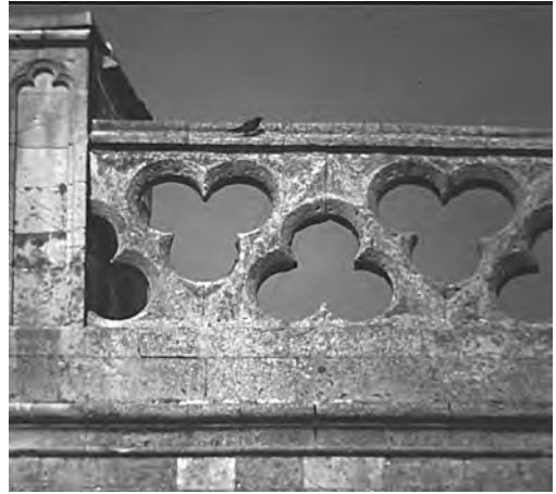
Fig. 17 Keynsham parish church tower parapet
