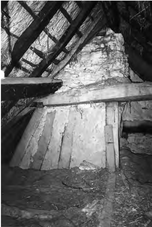
Fig. 4 Bramble Cottage, Haselbury Plucknett, smoke-hood
