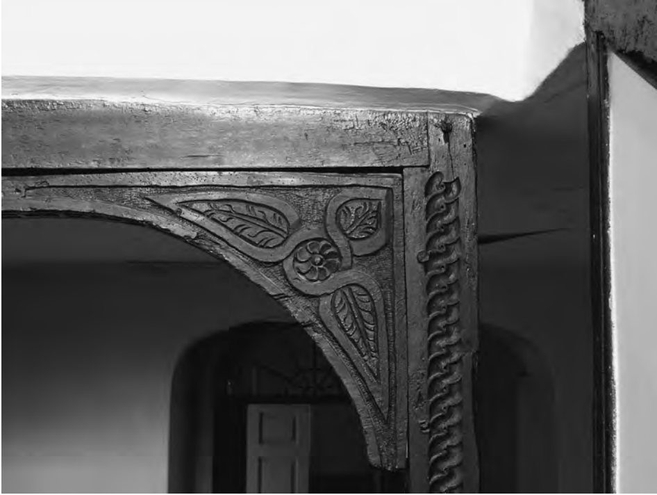
Fig. 9 Tintinhull House, spandrel at foot of back stair
