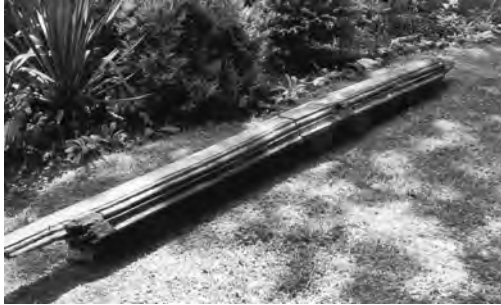
Fig. 8 Ile Cottage, Combe St Nicholas, moulded beam removed during the raising of the ceiling height; photograph John Rickard
