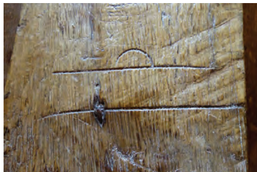
Fig. 7 Misterton, Newberry Lane, Dry Close: carpenter's mark for 2 on partition post
