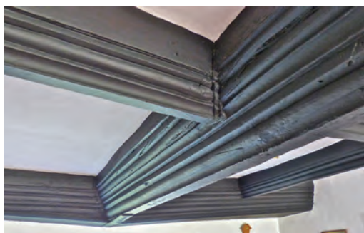
Fig. 1 Ashill, Southtown Farm: 16 th century framed ceiling, two orders of framing
