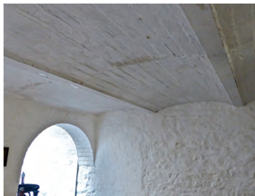
Fig. 2 Bruton, 27 High St: iron-beamed, brick-vaulted, fire-proof ceiling
