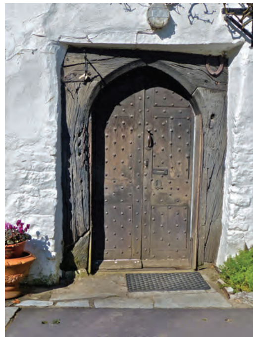
Fig. 10 Rimpton, Clarkes Cottage: early 15 th -century door frame
