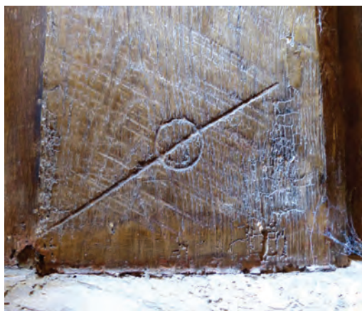
Fig. 6 Misterton, Newberry Lane, Dry Close: carpenter's mark for 1 on partition post
