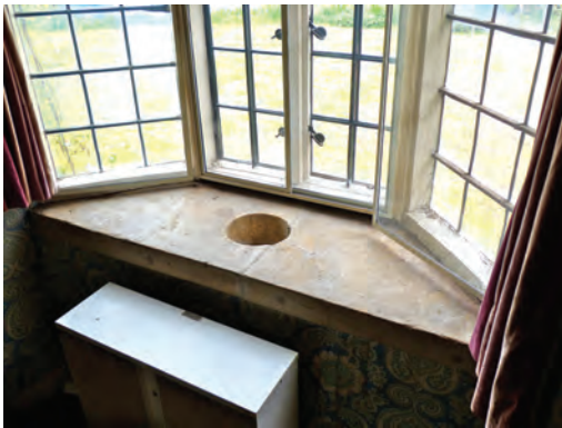
Fig. 9 Queen Camel, Banksia; "stewing stove" in window bay
