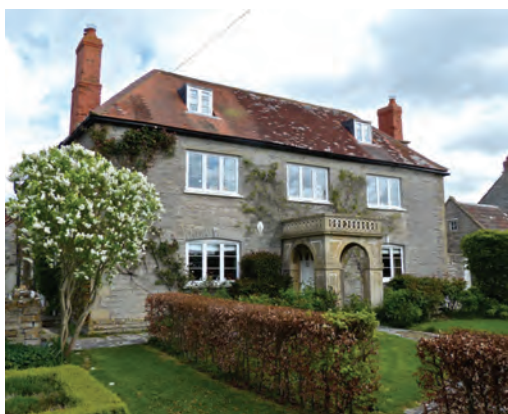
Fig. 3 Ditcheat, Wraxall House: House dated 1811 and portico dated 1871
