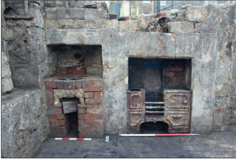
Fig. 5 Detail of fireplace with iron range (right) and later oven with 'copper' (left) at Plot 4 Bridewell Lane, looking south (scales 0.5m and 1m)
