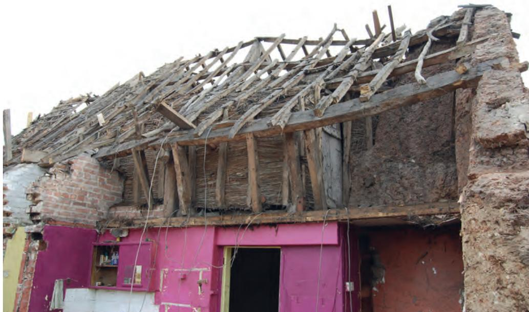
Fig. 7 Rear showing small room with door alongside cob chimney, cob gable wall, additional supports to lower purlin, and later first floor internal stud wall of reed and plaster (looking E)
