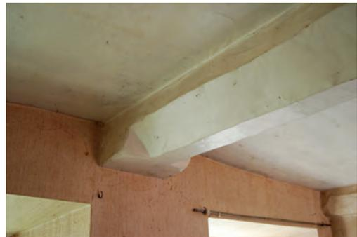
Fig. 6 Bridging beam showing steep chamfers and square stop
