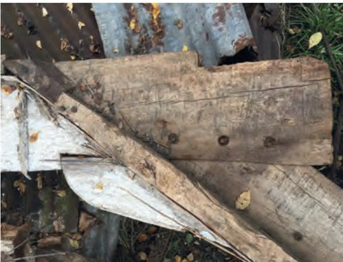
*Fig. 3 Side-pegged long-tenon joint of Truss 2 following removal*
