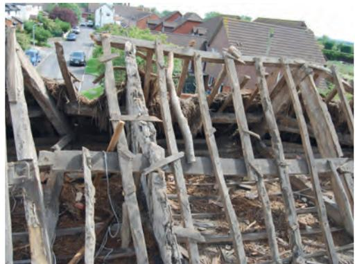
*Fig. 4 Truss 1 and 2 with collars, and purlin with splayed scarf joint and dovetail joint (looking SE)*
