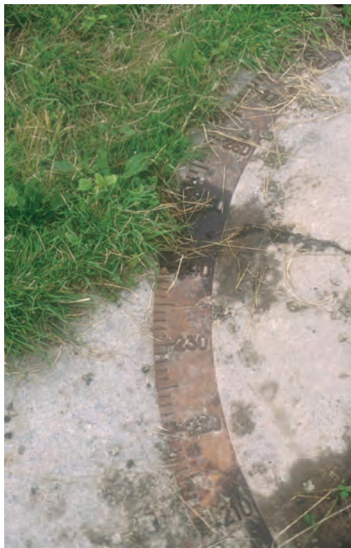
Fig. 5 Detail of the iron protractor ring on Base 16 in 1998. Somerset HER image 652.
