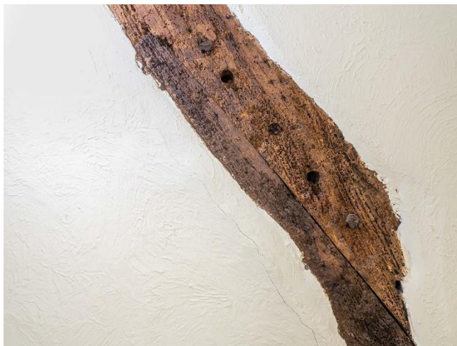
A Dunster Example of a Jointed Cruck Blade
