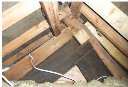
Fig. 8 Porlock, Ye Old Cottage: apex of jointed cruck frame
