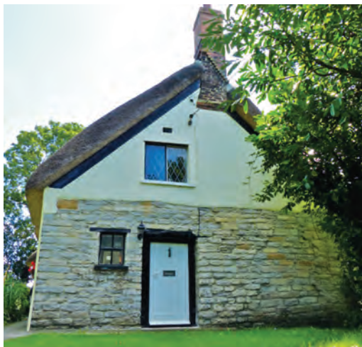
Fig. 7 Kingsbury Episcopi, Thorney, The Anchorage, west entrance into inglenook
