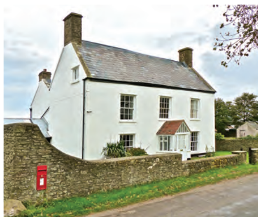
Fig. 1 Clevedon, Dowlais Farm, south frontage
