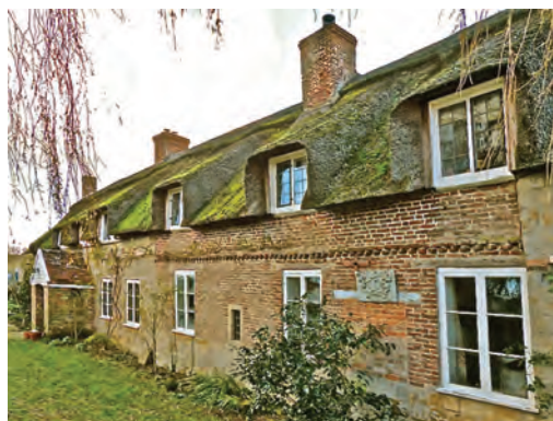
Fig. 12 Stocklinch, Ilford Bridges, front elevation displaying decorative brickwork
