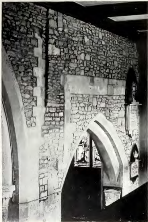
FIG. 1.—MASONRY AT E. END OF S. AISLE.
