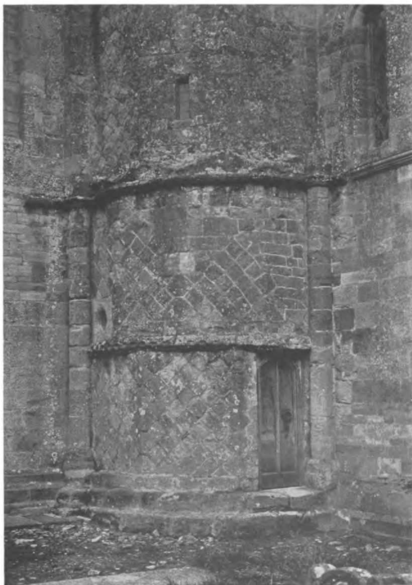
CHURCH OF ST. JOHN THE EVANGELIST, MILBORNE PORT. The three lower stages of the Stair Turret, of Norman date.
