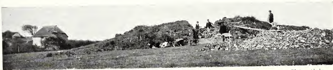
FIG. 3.—View from the E.S.E., showing the eastern cutting.
