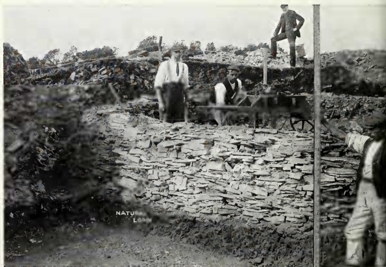
FIG. 2.—View of the south face of the Wall, showing the natural loam on which it was built.
