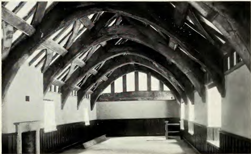
THE ROOF OF THE CHURCH HOUSE, CROWCOMBE.
