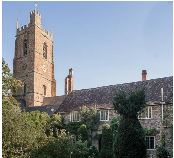
Priory Farmhouse Exterior - N elevation Copyright A. Harding
