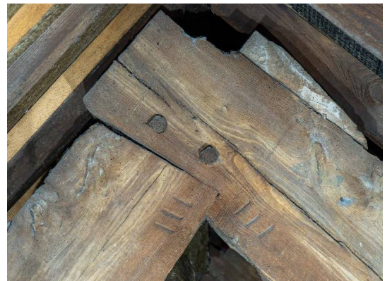
Marks (III) cut with a chisel
