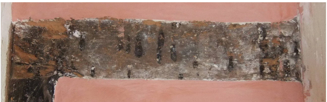
Marks on (top) fireplace bressumer and (above left and below) wall framing
