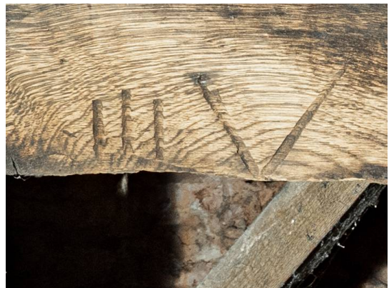
Marks (IIIV) made by gouging
