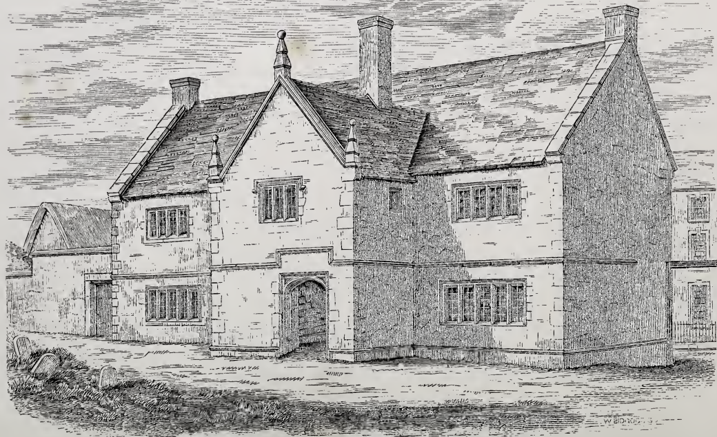
THE SOUTH FRONT OF THE GRAMMAR SCHOOL, CREWKERNE.
