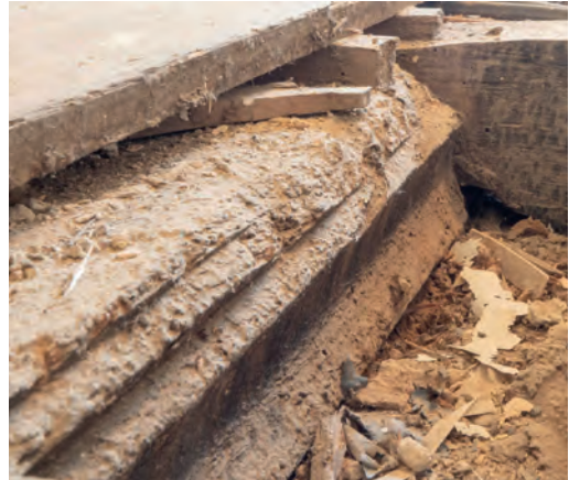
Fig. 10 Profile of assumed jetty beam b3
