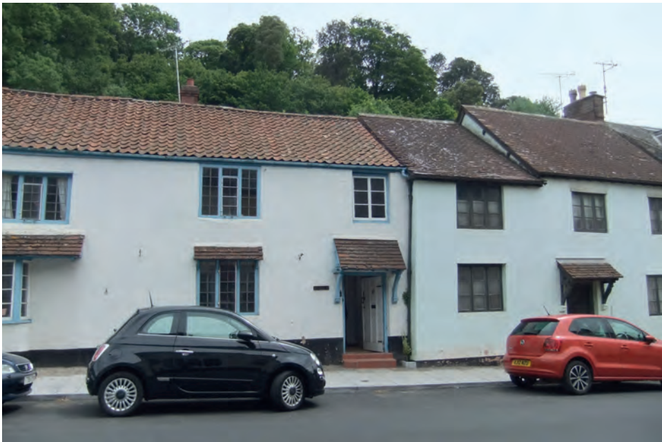
Fig. 8 Line of roof extending south under a different roof finish (at right of photograph)
