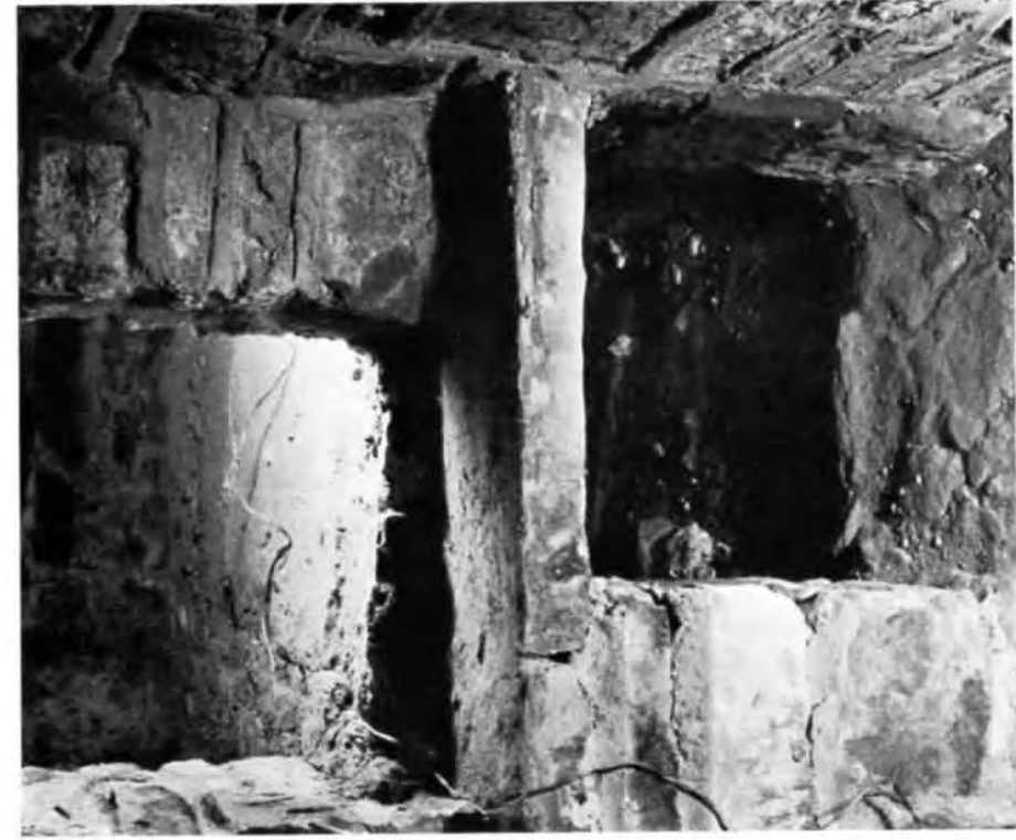
Plate 1. Floor of oven inserted above earlier hearth tunnel to bacon chamber at Stoneley Farm, Kingsdon.
