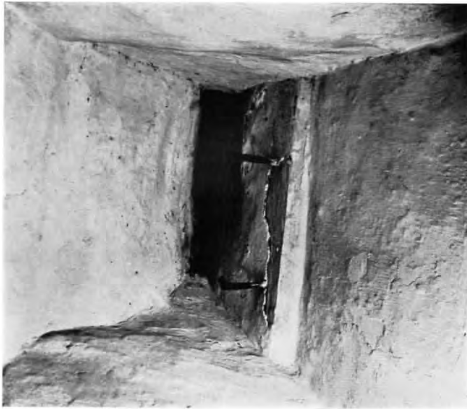
Plate 4. Return flue from top of type 4 fully enclosed chamber at Fir Tree Farm, Low Ham, with bacon hooks still in situ.
