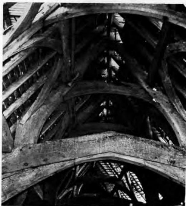
Glastonbury Abbey Barn Upper cruck standing on the tie beam
