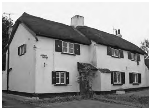
Fig. 15 Winscombe, Orchard Cottage (photo John Rickard)
