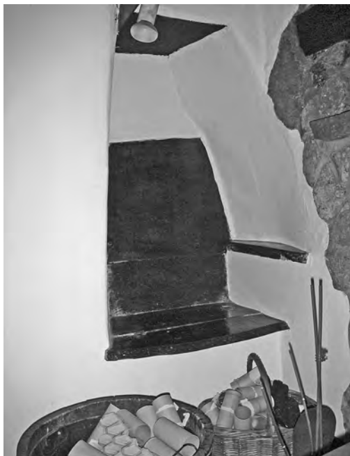
Fig. 14 Winscombe, Yew Tree Farm and Cottage (photo Mike Hargreaves)
