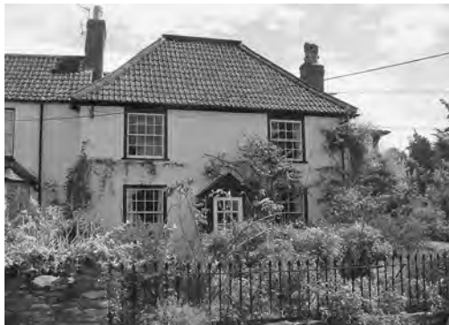
Fig. 19 Winscombe, Harbury Batch (photo John Rickard)
