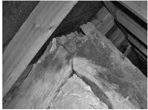
Fig. 13 Winscombe, Laurel Farm, apex of roof principals (photo John Rickard)
