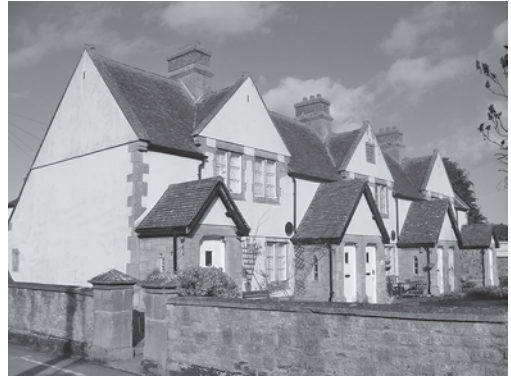
Fig. 4 Stogursey, Lime Street almshouses (photo Mike Hargreaves)
