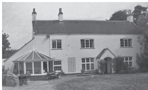
Fig. 19 Winscombe, Sandford House, south elevation (photo Mike Hargreaves)
