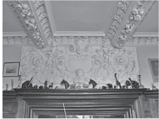
Fig. 8 Stogursey, Steyning Manor South. Ornate plasterwork on overmantel and ceiling beams (photo, John Rickard)
