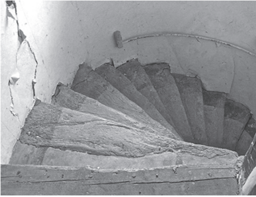
Fig. 7 Stogursey, Baulk timber stair at Steyning Manor North (photo John Rickard)
