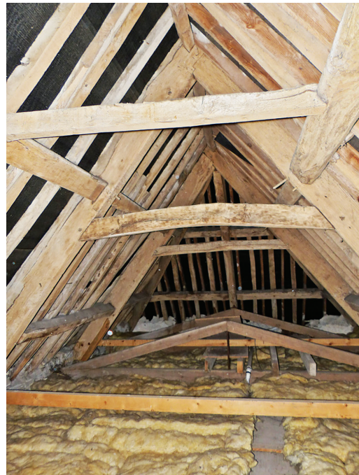
Fig. 3 Doultong, King's Rd, Hurlingpot Farmhouse, the roof trusses and the shallow hoist truss
