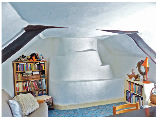
Fig. 12 Wambrook, Beechwood, rounded and stepped stack at first floor level
