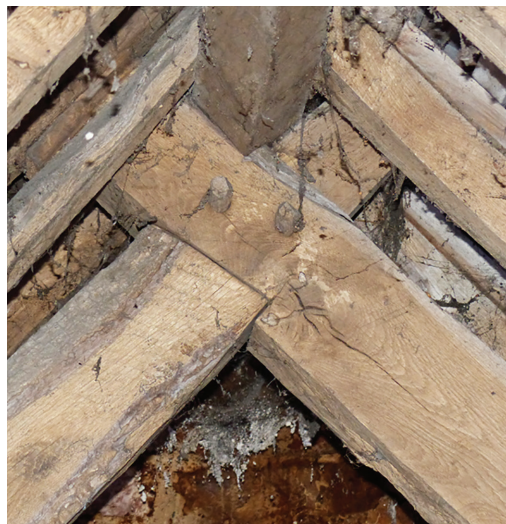
Fig. 13 Devon, Tytherleigh, Chard Rd, Penny Cottage & 2, Pinney Cottage, the halved and pegged truss apex
