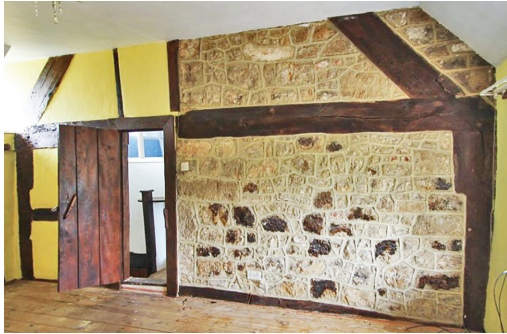
Fig. 2 Donyatt, Chard Rd, Thatchers Pond Frame FIII and truss with masonry replacing a possible fire hood of wattle and daub
