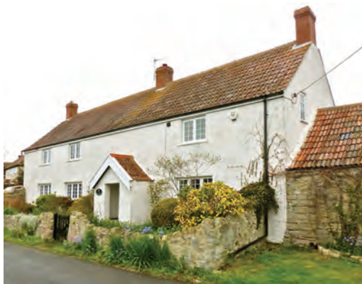
Fig. 8 Pawlett, 14 Gaunts Rd, Doidges House, south elevation
