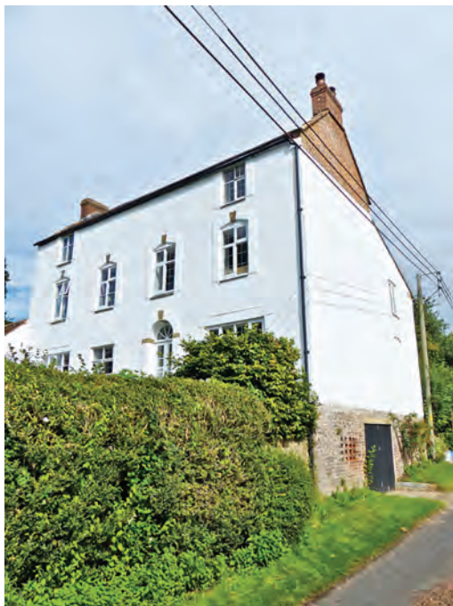
Fig. 6 Kingsbury Episcopi, Mid Lambrook, The White House, south-east elevation
