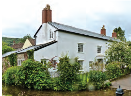
Fig. 1 Burrington. Rickford, Brook House from NE
