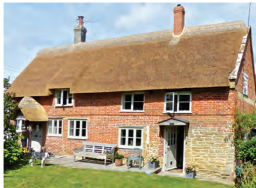
Fig. 5 Kingsbury Episcopi, East Lambrook, Townsend Cottage, south elevation
