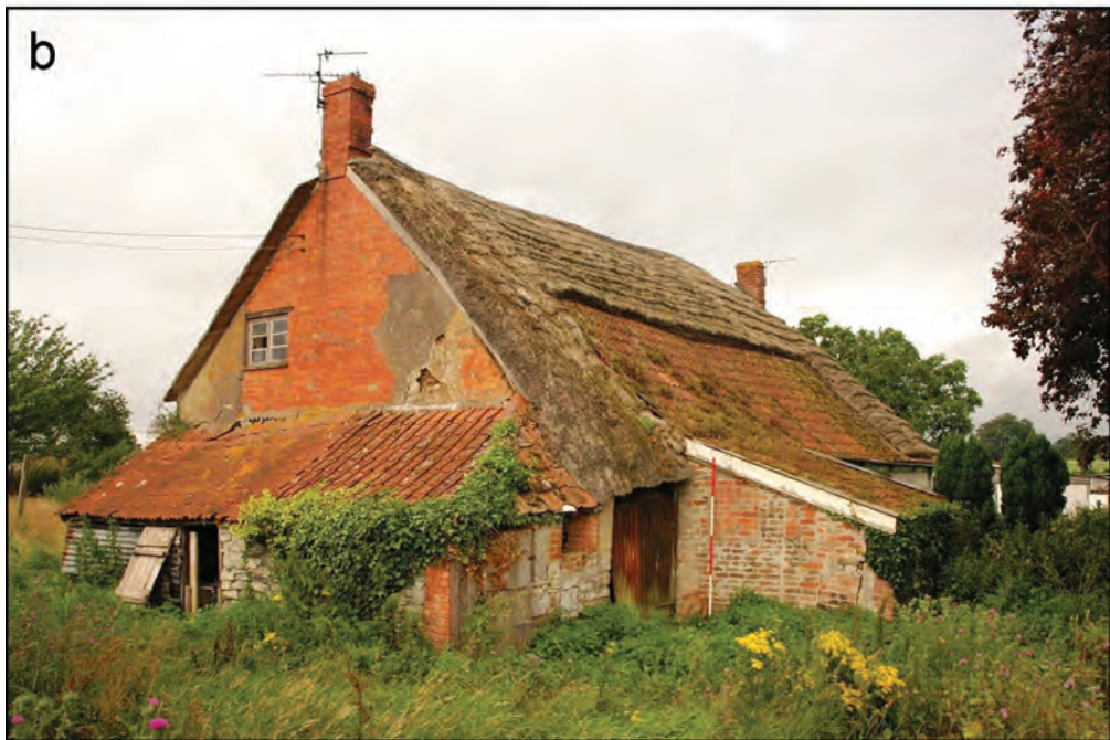
Fig. 1 Broad Lane Farmhouse. (a) From the lane to the north, showing the extent to which the early house is concealed by later outshuts and extensions. (b) From the south-east, showing the gable end rebuilt in brick (photos: Gary Young)
