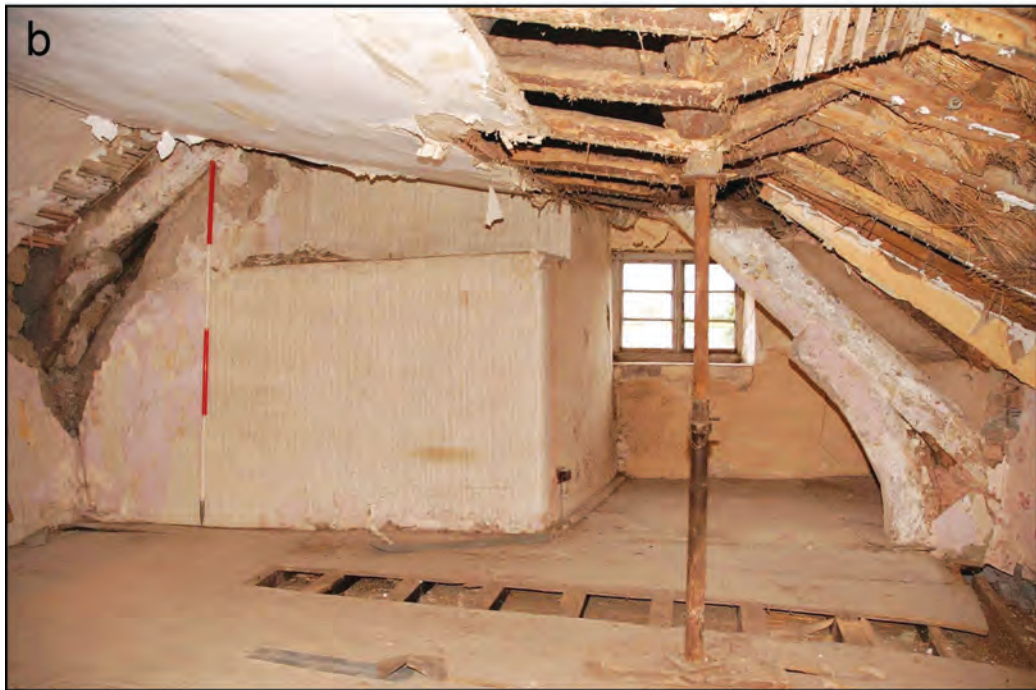
Fig. 8 (a) Section I: the south-eastern end of the house, showing the character of the roof truss over the hall, the inserted fireplace behind it and the extent to which the roof has sagged (based on hand-measured survey by Exeter Archaeology). (b). View at first-floor level (photo: Gary Young)
