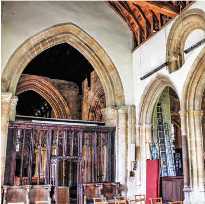
*Fig. 22 Northwest angle of the chancel with original arch reset into the upper north wall*
