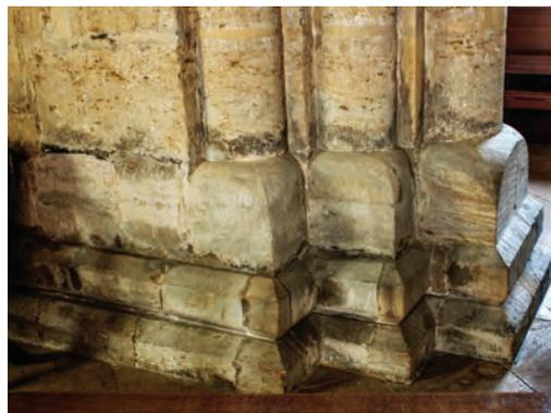
*Fig. 16 Inverted cushion bases, west responds of north crossing arch*
