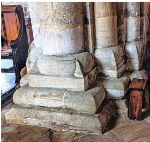
*Fig. 15 Bulbous bases with spurs, north responds of western crossing arch*
