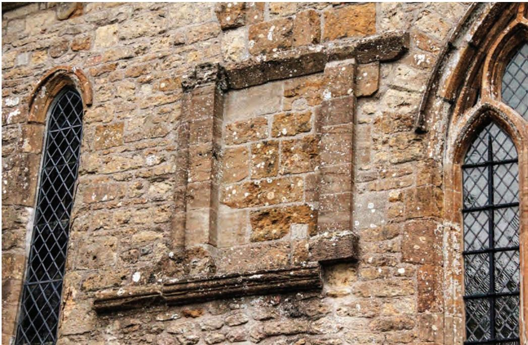
*Fig 12 Detail of the engaged column positioned adjacent to a pilaster on the south chancel wall*
