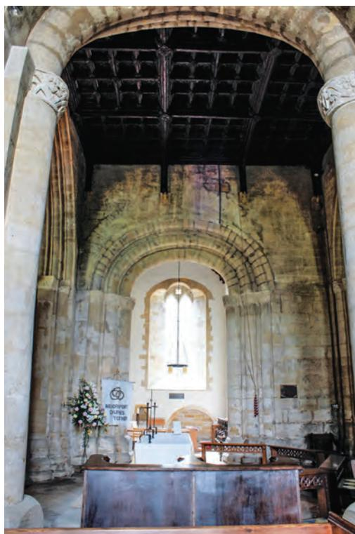
*Fig. 8 South crossing arch showing the wider western wall at the location of the external stair turret*
