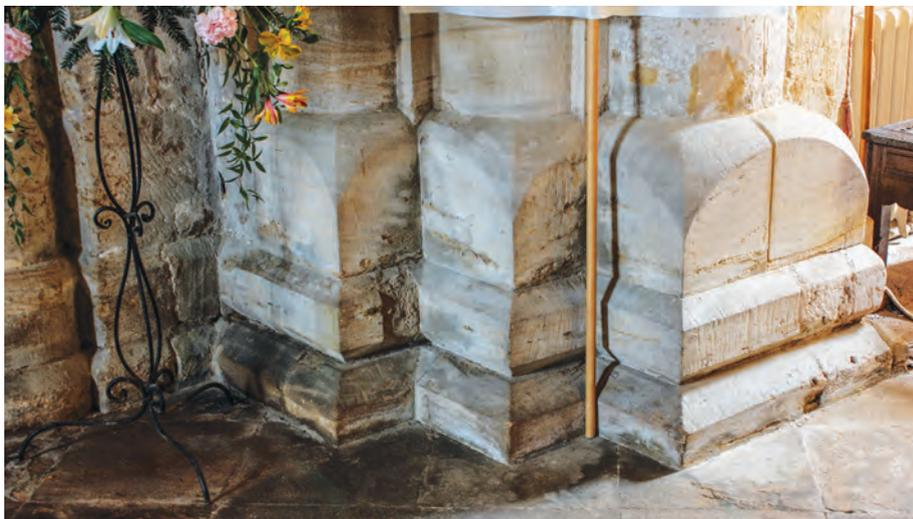
*Fig. 7 Detail, inverted cushion bases, east responds of south crossing arch*
