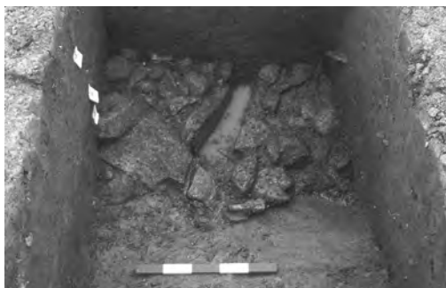
Fig. 22 Site 1, stone-lined culvert 328; view south
