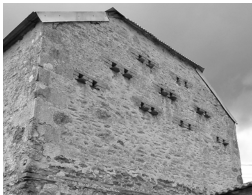
Fig. 13 Pairs of brick nest-holes in the gable end of a stone barn at Tirelands Farm, Enmore (photo Somerset Vernacular Building Research Group)
