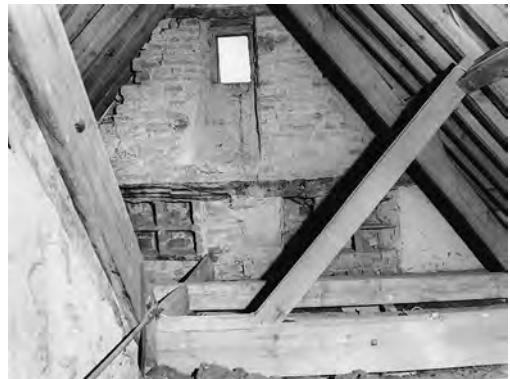
Fig. 11 The Manor House, Marston Magna. The nest-boxes formed in a blocked window on the second floor of the rear range (photo John McCann)
