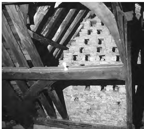
Fig. 9 Nest-holes in the south gable of the medieval hall, Birdcombe Court, Wraxall (photo John McCann)
