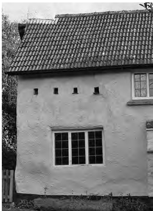
Fig. 12 Nest-holes in an ancillary building of Troyte's Farm, Tivington in Selworthy (photo J.C. Bond)
