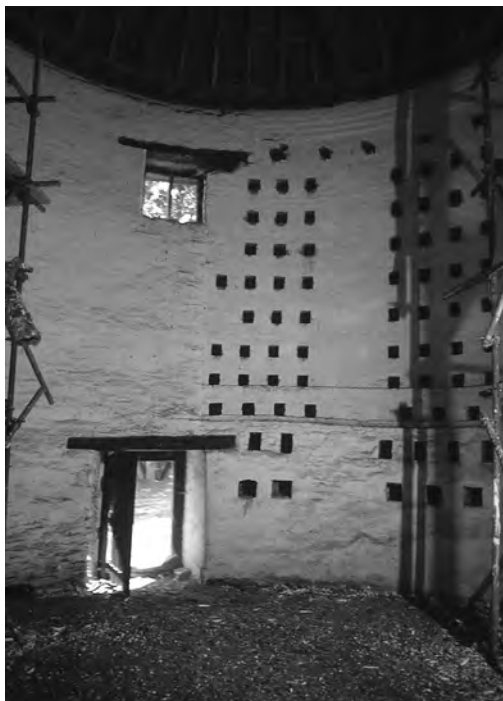
Fig. 5 Halswell House, Goathurst. The interior, facing east. The plinth and doorway are original. The east window has a charred frame and lintel (photo John McCann)
