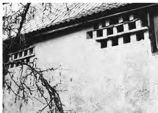
Fig. 10 Nest-holes in the south elevation of the medieval range of Steyning Manor, Stogursey (photo John McCann)
