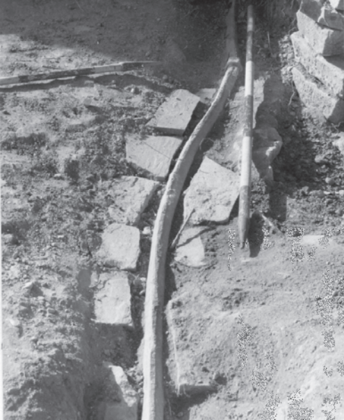
Fig. 9 Vestibule: lead piping under floor; view north
