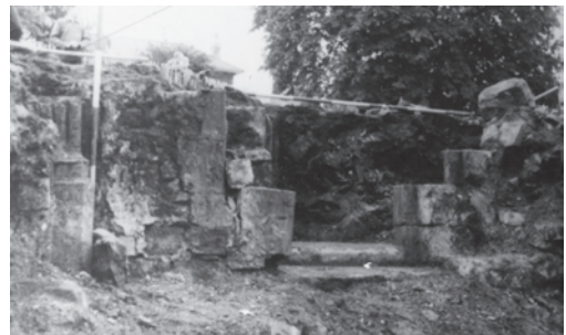
Fig. 17 Doorway to possible infirmary; view south
