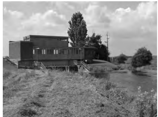
Fig. 1 The pumping station at West Moor
