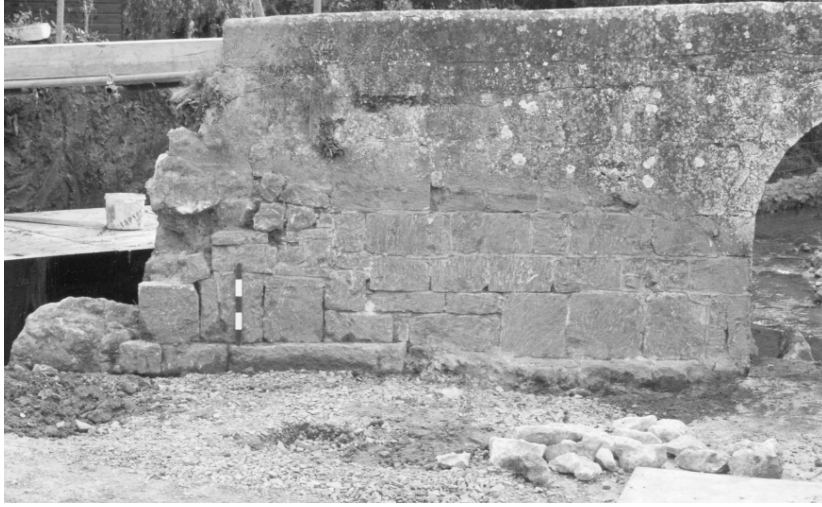
Fig. 4 South end of bridge, 0.5m scale stands on base course of Period 1 bridge; view west
