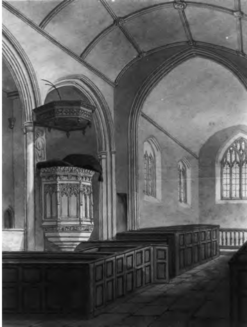
Fig. 4 Worle Church, 1829, by J.C. Buckler, including box pews, pulpit, pulpit cushion, sounding board, altar rail and ribbed wagon roof
