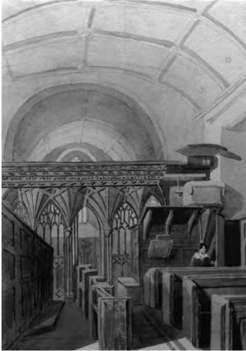
Fig. 3. St Audries Church, West Quantoxhead, 1845, by S.G. Tovey, including ribbed wagon roof, rood screen, box pews and bench seats, pulpit with sounding board, reading desk and (possibly) clerk's desk
