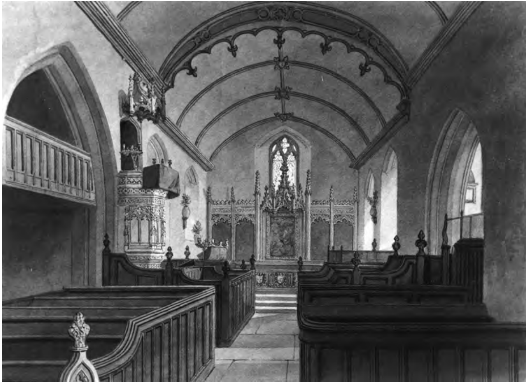
Fig. 1. Brockley Church, 1829, by J.C. Buckler, including gallery in north aisle
