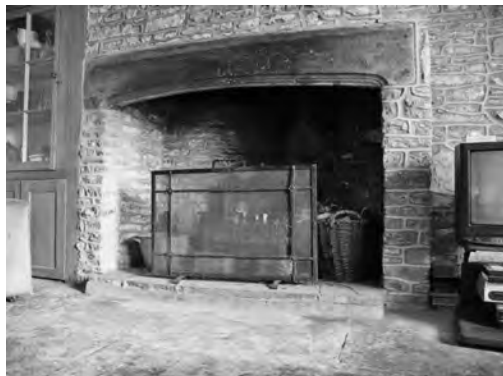
Fig. 3 Gilcombe House, Blagdon, fireplace with moulded bressumer
