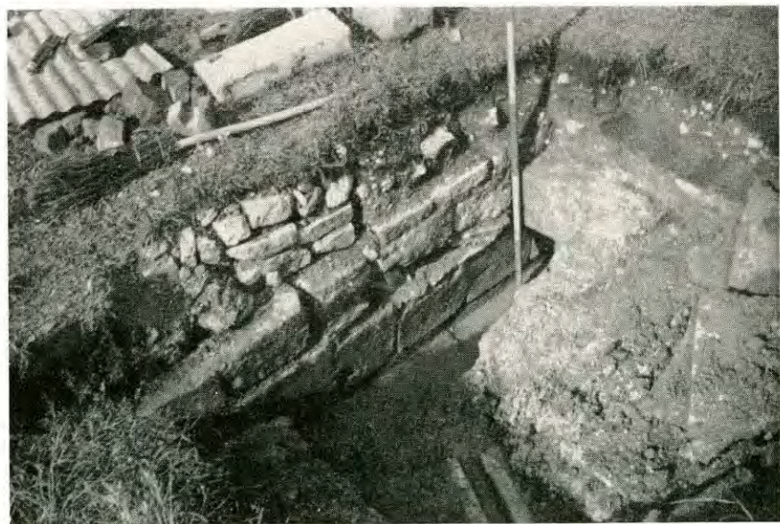
(b) WATER CONDUIT UNDER N.W. CORNER OF CELL 14. TAKEN FROM S.W.
