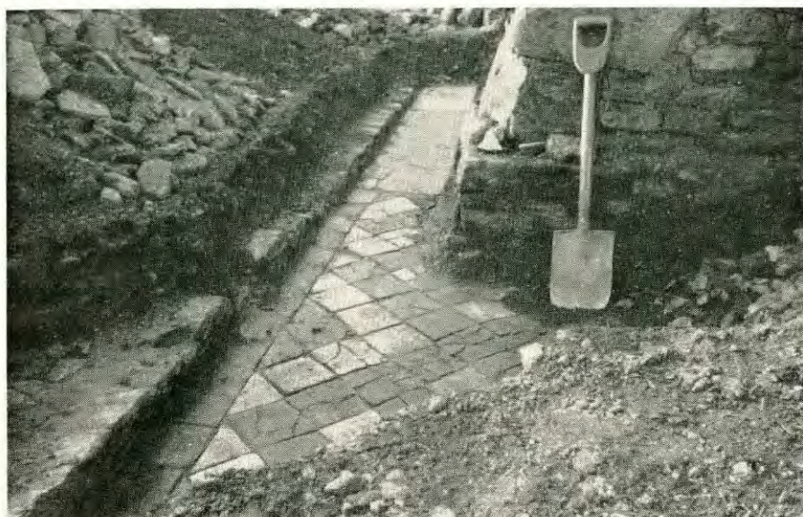
(a) CLOISTER ALLEY AND PENTICE WALL ON SOUTH SIDE OF REFECTORY. TAKEN FROM EAST
