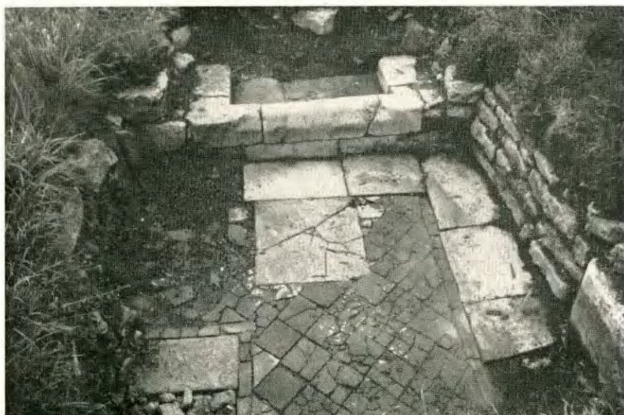
(b) N.W. CORNER OF CLOISTER ALLEY AND ENTRANCE TO CELL 14. TAKEN FROM EAST
