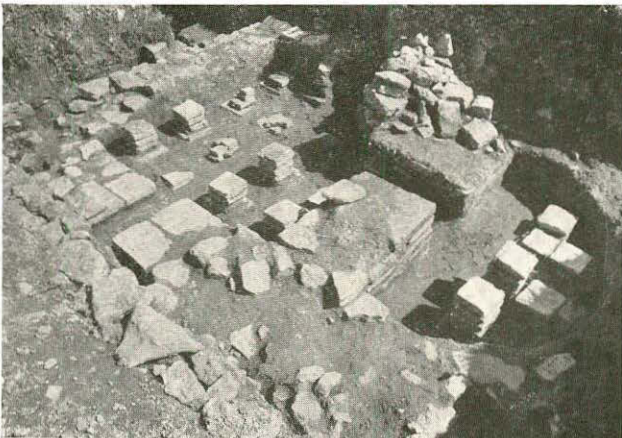
2. Hypocaust of Rooms 10 and 11 from N.W.
