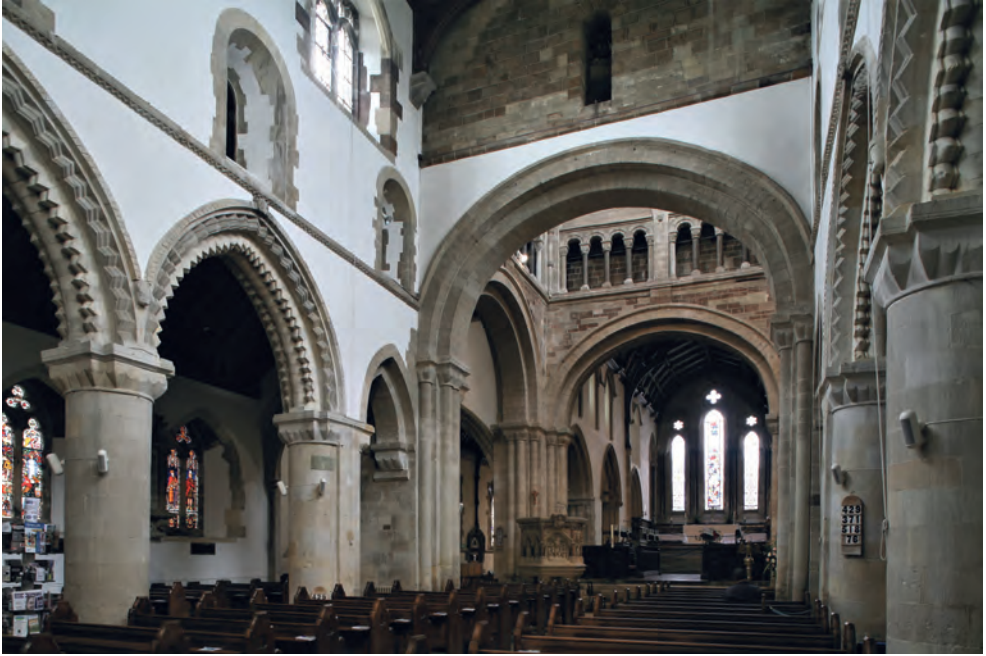
Fig. 5 Wimborne Minster, interior to E from nave
