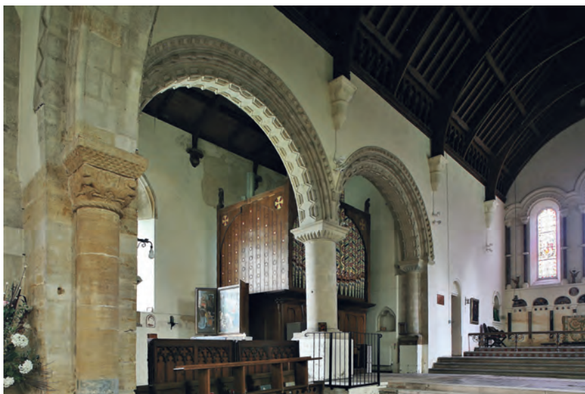
Fig. 22 Stogursey, St Andrew, presbytery, interior to NE
