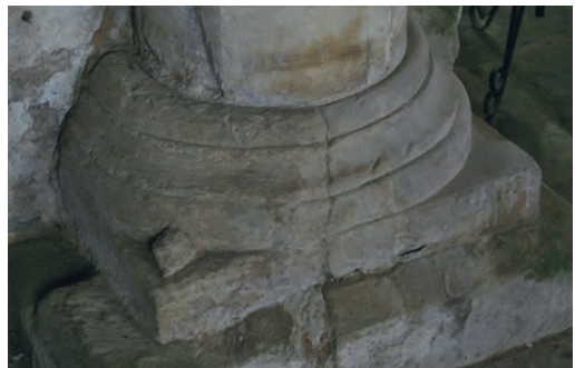
Fig. 19 Stogursey, St Andrew, E crossing arch, S respond base
