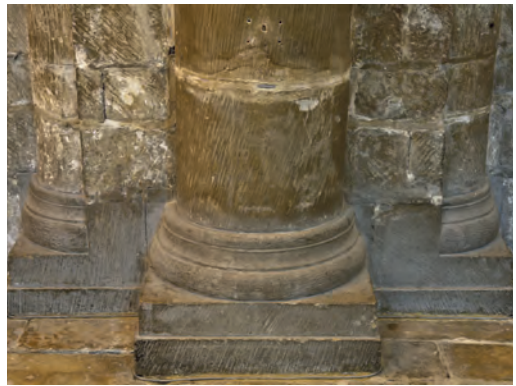
Fig. 18 Gloucester, St Peter's abbey, N nave aisle, detail base
