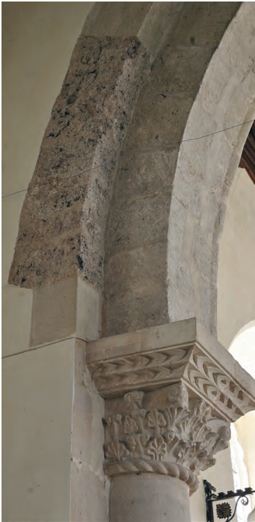
Fig. 20 Stogursey, St Andrew, crossing to SW detail
