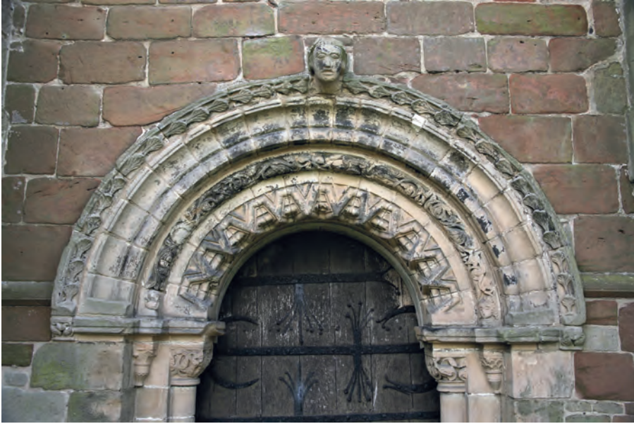
Fig. 37 Edstaston (Shropshire), St Mary, N nave doorway
