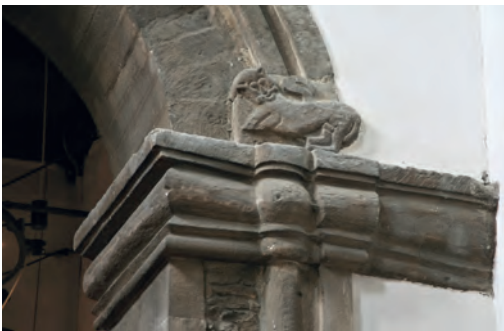
Fig. 16 Cambridge, St Bene't, arch from nave to W tower, N capital
