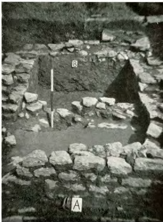
ROOM 10. (A) LEAD WASTE-PIPE. (B) STUCCO LINING BELOW FLOOR LEVEL.
